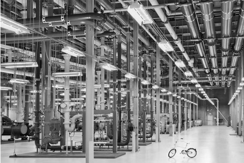
**Figure 3.1.** Douglas County, Georgia, data center. Shown here are colorful pipes distributing water for cooling the facility, and Google's G-bike, the "vehicle of choice" for transportation in and around the data centers.
