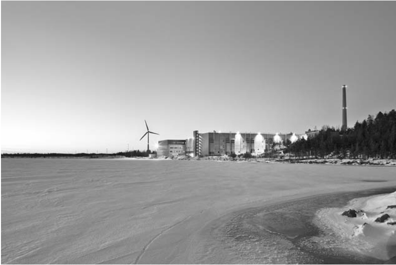
Figure I.1. A Google data center sits in the icy landscape of Hamina, Finland, where system operation is more energy efficient.
