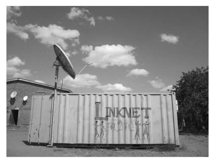
Figure 5.2. Machans could access the Internet from 2011 to 2012 from several LinkNet VSAT terminals built out of repurposed cargo containers. Photo by author.
